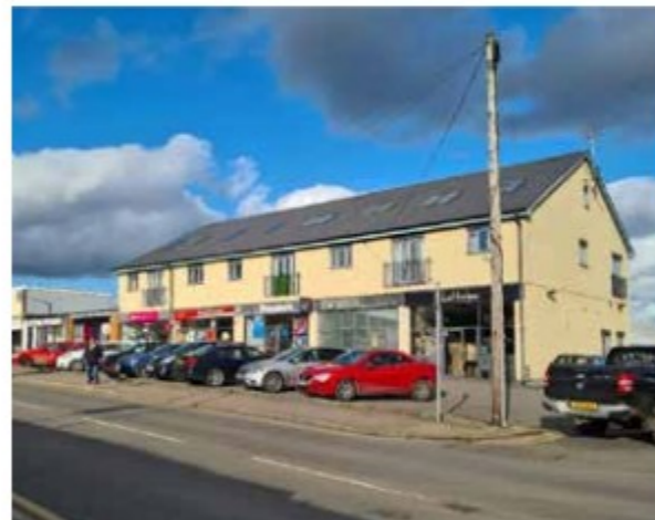
Bulwark shops neighbourhood centre
