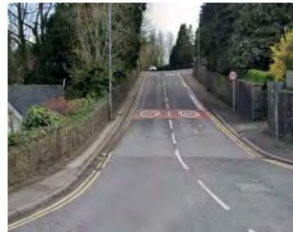
Narrow footways on busy road
